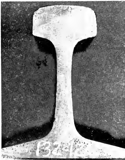
Fig. 6 (Investigation 132-12A)—Cross section of a rail that was cut through a point exhibiting an internal imperfection. This imperfection, detected by a Sperry detector car and hand test, can be noted in the web.
